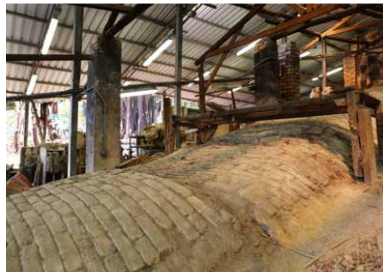
左 窯脊的一部分開始凹陷。 右 龍窯不同位置的截面，可見窯腔各處的大小變化。圖由工務局繪製。 L Part of the kiln spine has started to cave in. R Elevation drawing by the Public Works Department shows cross sections of the kiln interior.
